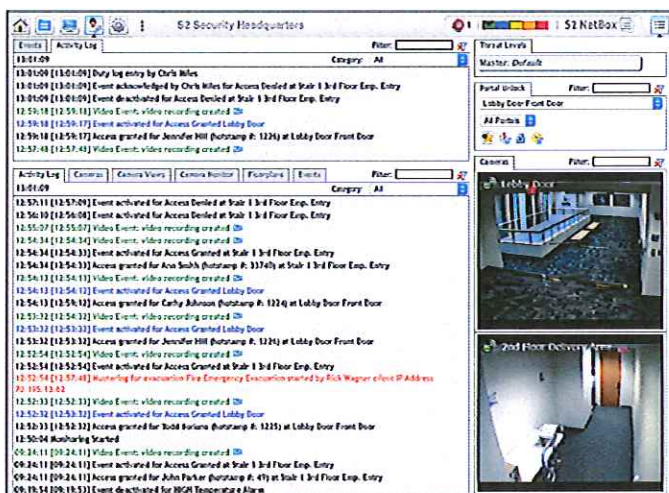
Access control and event monitoring for connected devices are aggregated to the S2 NetBox web interface.
